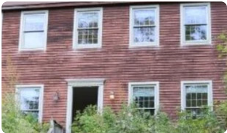
Photo 4. Windows and doors 1:04 PM
