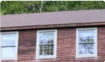
Photo 2. Roofline, from the ground 1:03 PM
